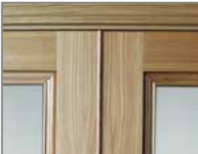
T-REBATE STRIP Our T-Rebate door slip is a convenient and stylish solution for double door installation.
